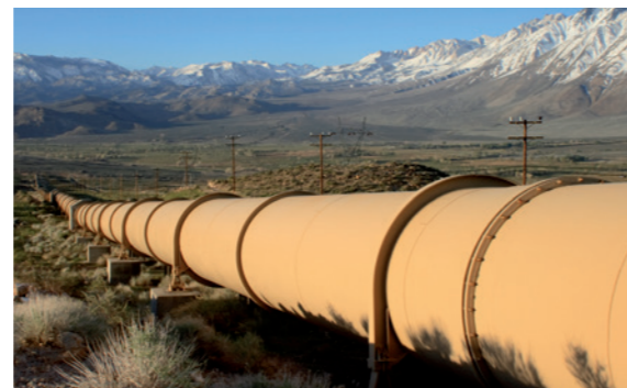
Testing the outer coating of a pipeline after a repair
